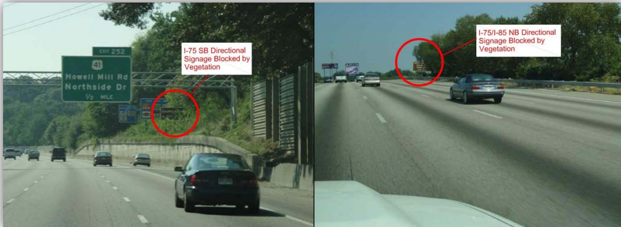
Figure 7-23. Samples of Interstate Directional Signs Blocked by Vegetation
